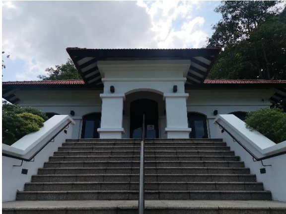
Exterior view of Raffles House
