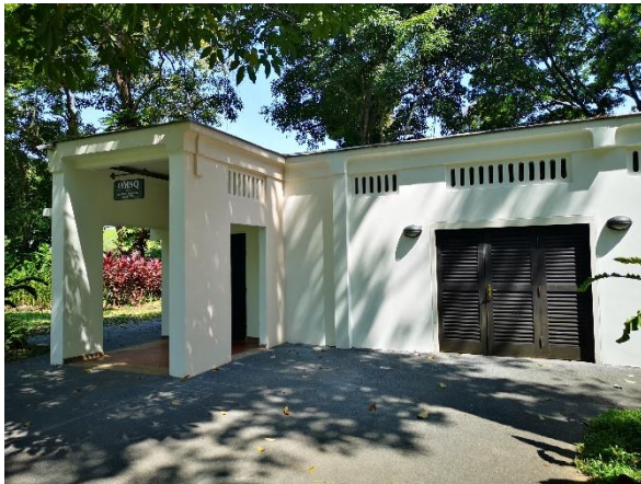
Exterior view of OMSQ
