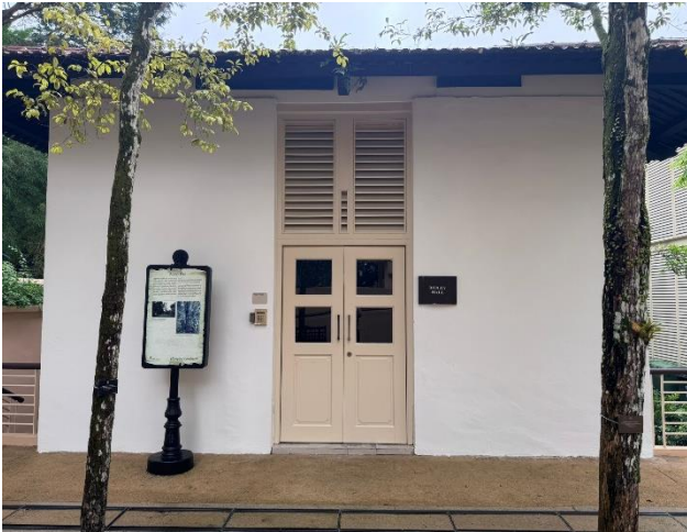
Exterior View of Ridley Hall
